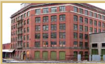
(Left to right) Historic Chancery Building and the Jensen-Byrd Warehouse
