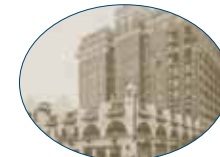
AUGUST Dallying at the Davenport DOWNTOWN DISTRICT, SPOKANE, WA • PAINTED OCTOBER 2008
